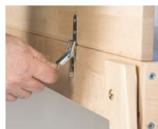
Fixing the guard rail to an upright position
